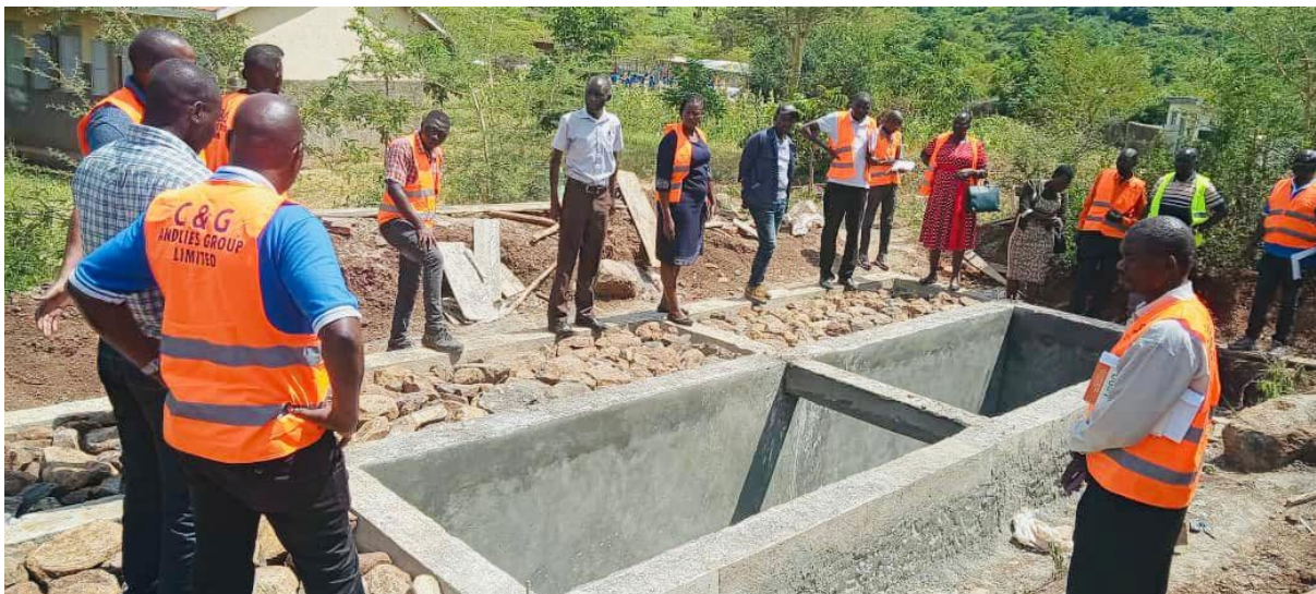
Building a model water reservoir, through Operation Wealth Creation Government of Uganda intends to do this around each homestead.
