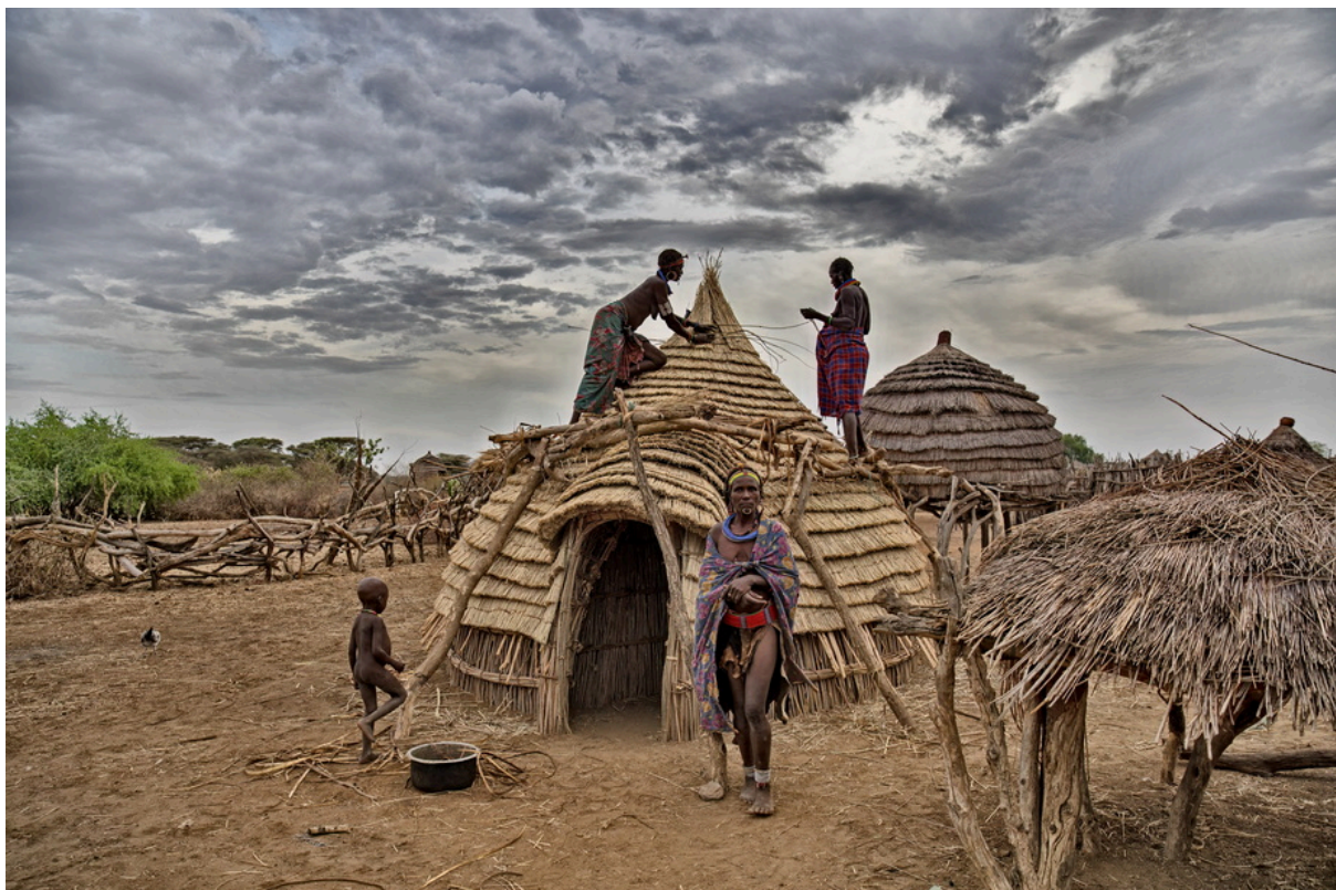
Toposa women repairing a traditional hut
